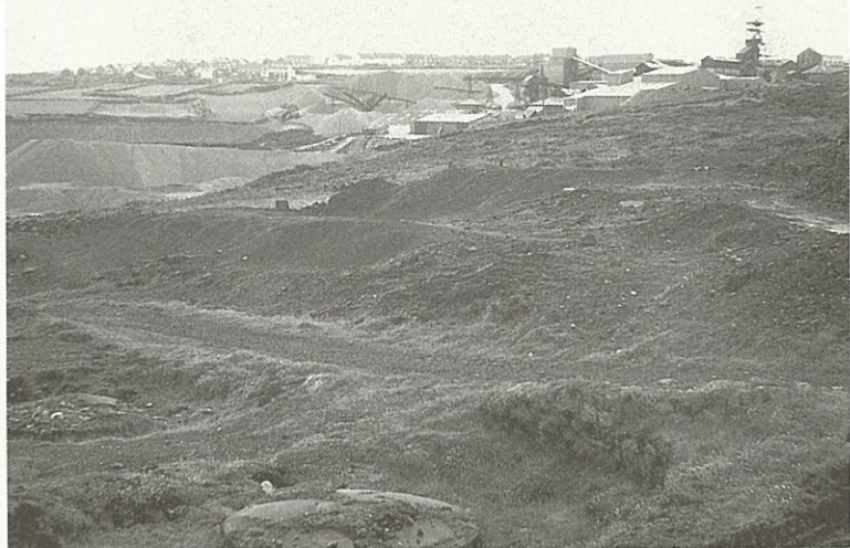
Plate 11 Geevor Mine: From left to right - stockpiled crushed aggregate, mill and headframe of Victory Shaft. In foreground, remains of round buddles formerly used for dressing of fine tin concentrate.
