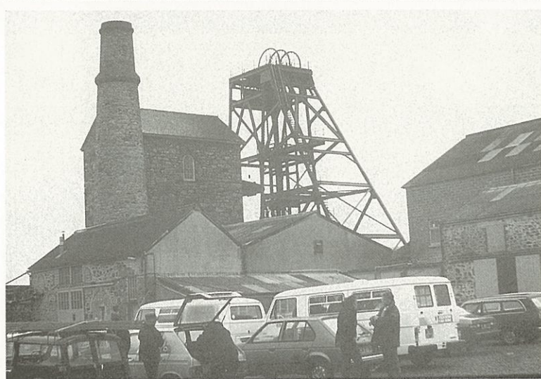
Plate 12 South Crofty Mine: Head-frame at Robinsons Shaft, 2021 feet deep, near Camborne. Robinsons 80-inch Cornish pumping engine with its 38 ton bob, built in 1854, was the last to operate on a mine (1903-1955).
