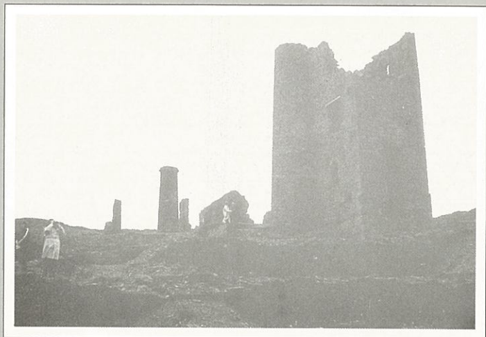
Plate 45 Stamps engine house and winder house (background) on the cliffs at Wheal Coates, Chapelporth, above Townroath Shaft. The Engine-house was built of killas in 1872.
