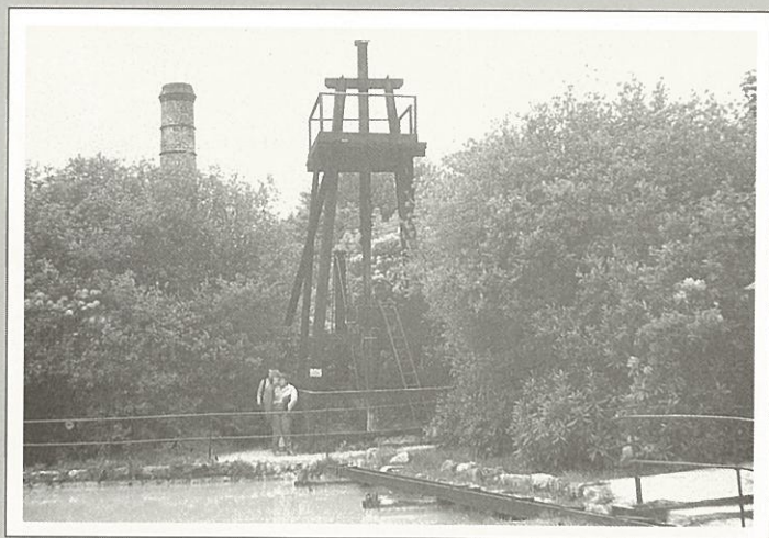
Plate 31 Wheal Martyn: Pump powered by waterwheel with clay settling tanks in foreground.
